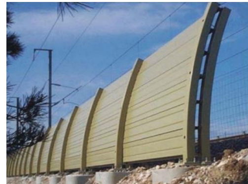
Noise Barrier, SNCF High Speed Train System, France
