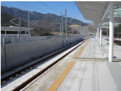
Noise Barrier, KTX High Speed Train System, Korea
