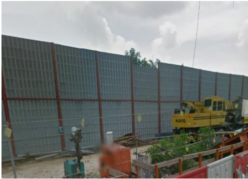
Temporary Noise Barrier, MRT Construction Site, KL
