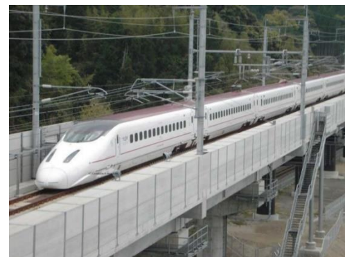
Noise Barrier, Japanese High Speed Train System
