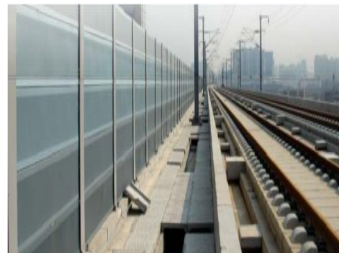
Noise Barrier, China High Speed Train System
